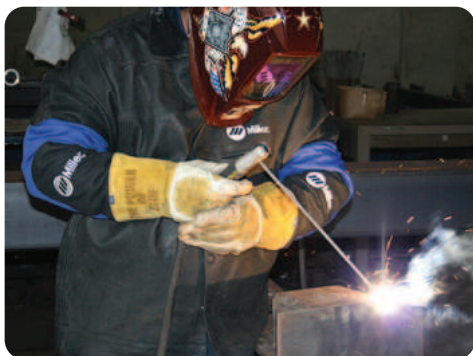
SMAW (Shielded Metal Arc Welding)
