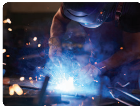
FCAW (Flux Core Arc Welding)
