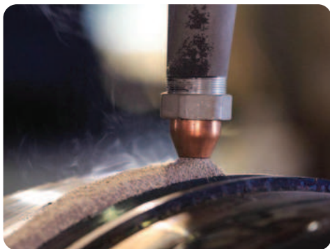
SAW (Submerged Arc Welding)
